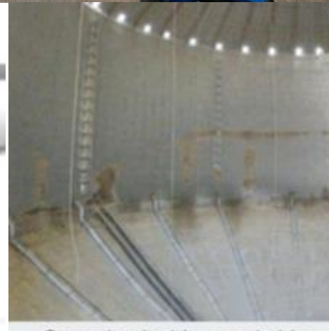
Corrosion inside a grain bin
